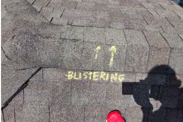
"Blistering," over time the asphalt shingles have begun to cook from inadequate roof ventilation.
