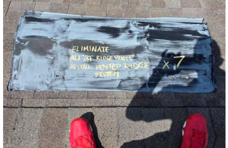
We will eliminate these static vents and install a vented ridge system to extend the new roof's life, as well as help to preserve the HVAC system and energy.
