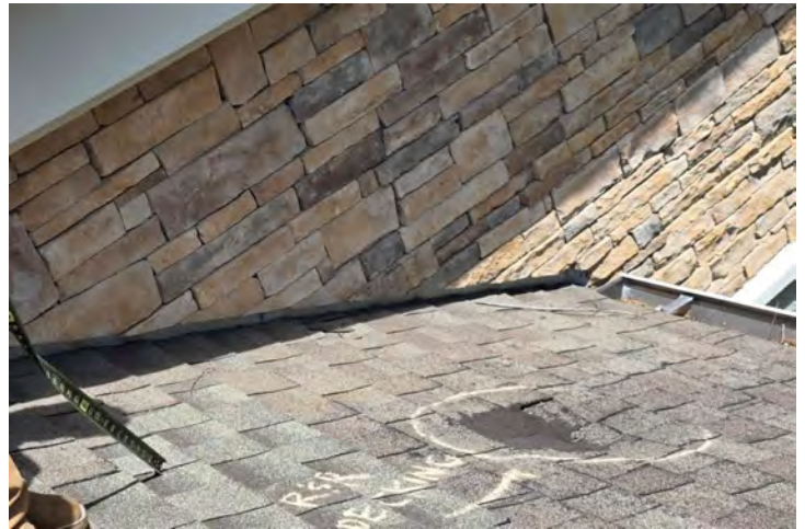
Projectile Damage
