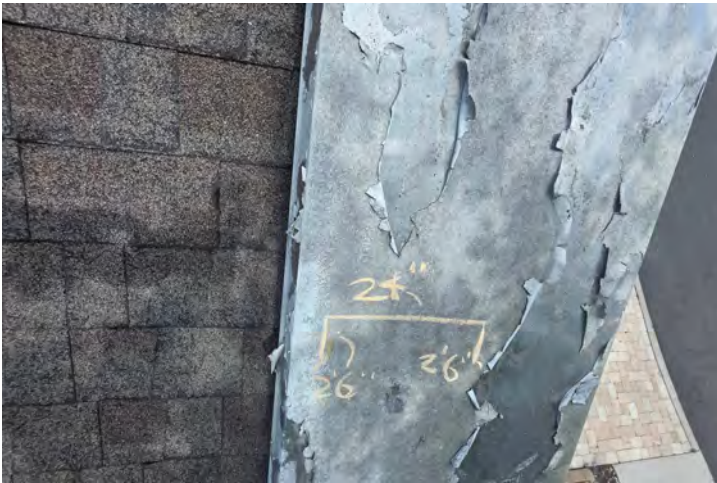
Front Porch Gable Wall Capping. Replace with Aluminum included (color TBD)
