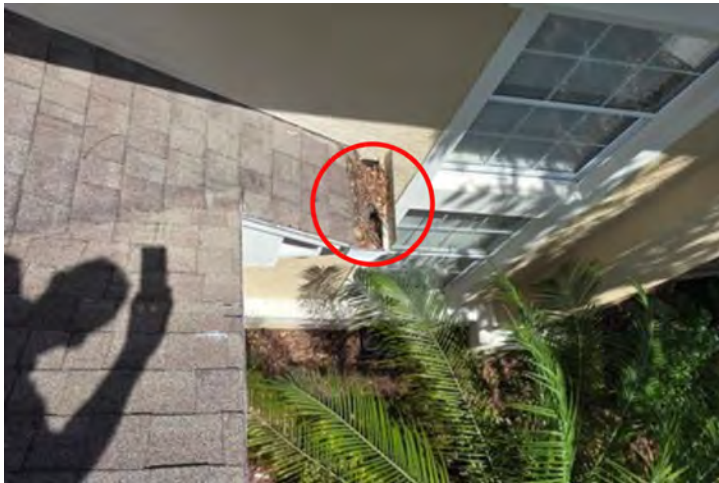
Gutters full. Gutter Guard upgrade option included
